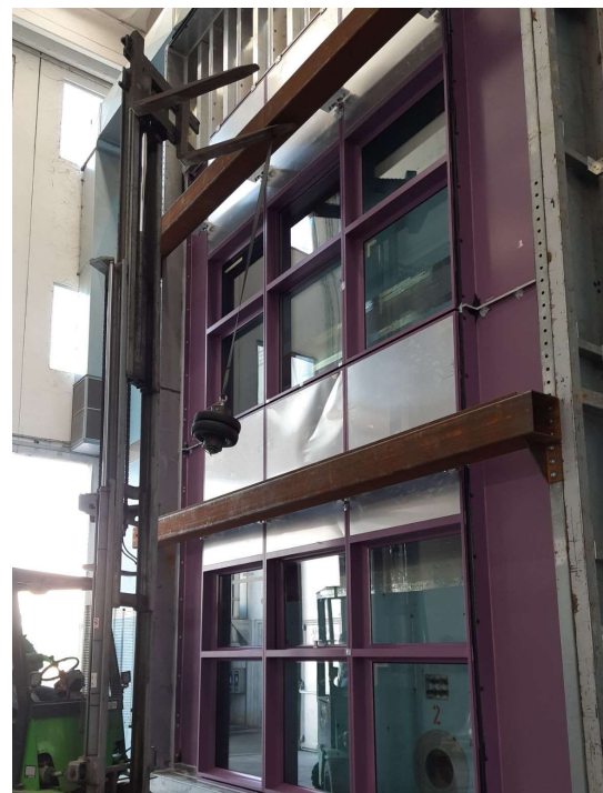
Figure 10 – Impact on the spandrel part top level in the metal sheet
