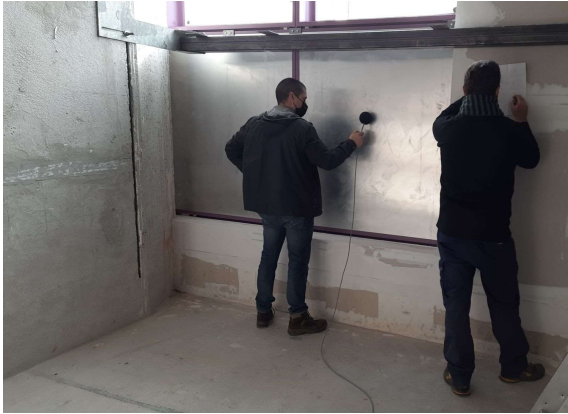
Figure 22 - Acoustic test - during the testing activities
