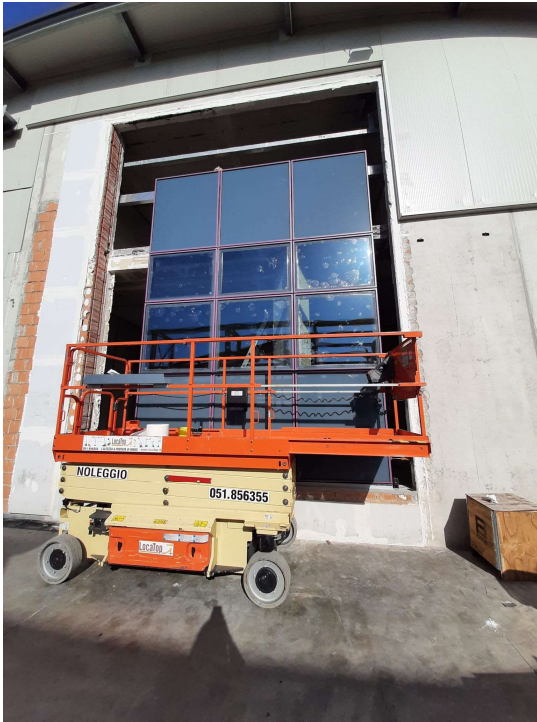
Figure 18 - Acoustic mock-up during the installation
