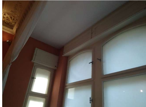
Figure 22: Polish Museum - Window view with old roller shutter boxes.
