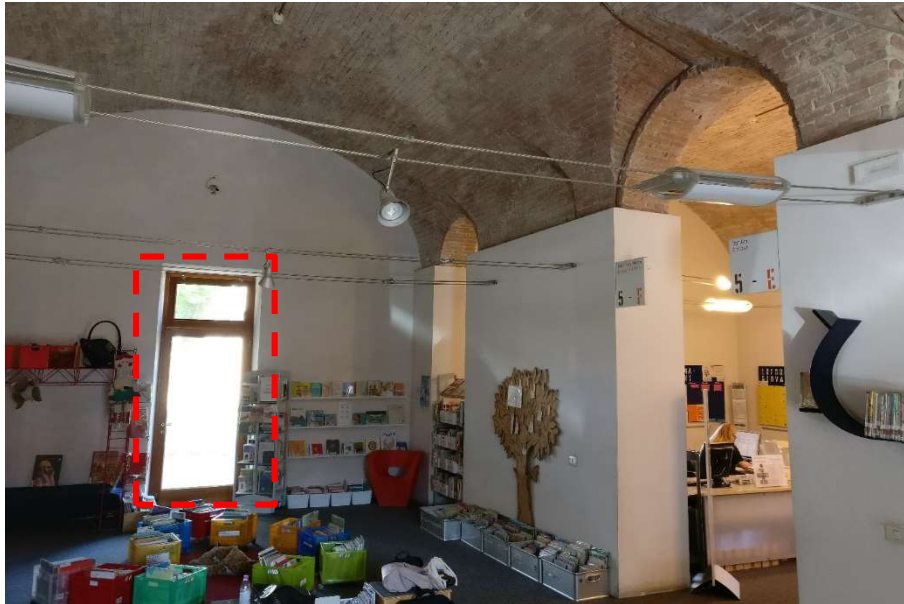
Figure 32 - San Giovanni Public Library: door-window
