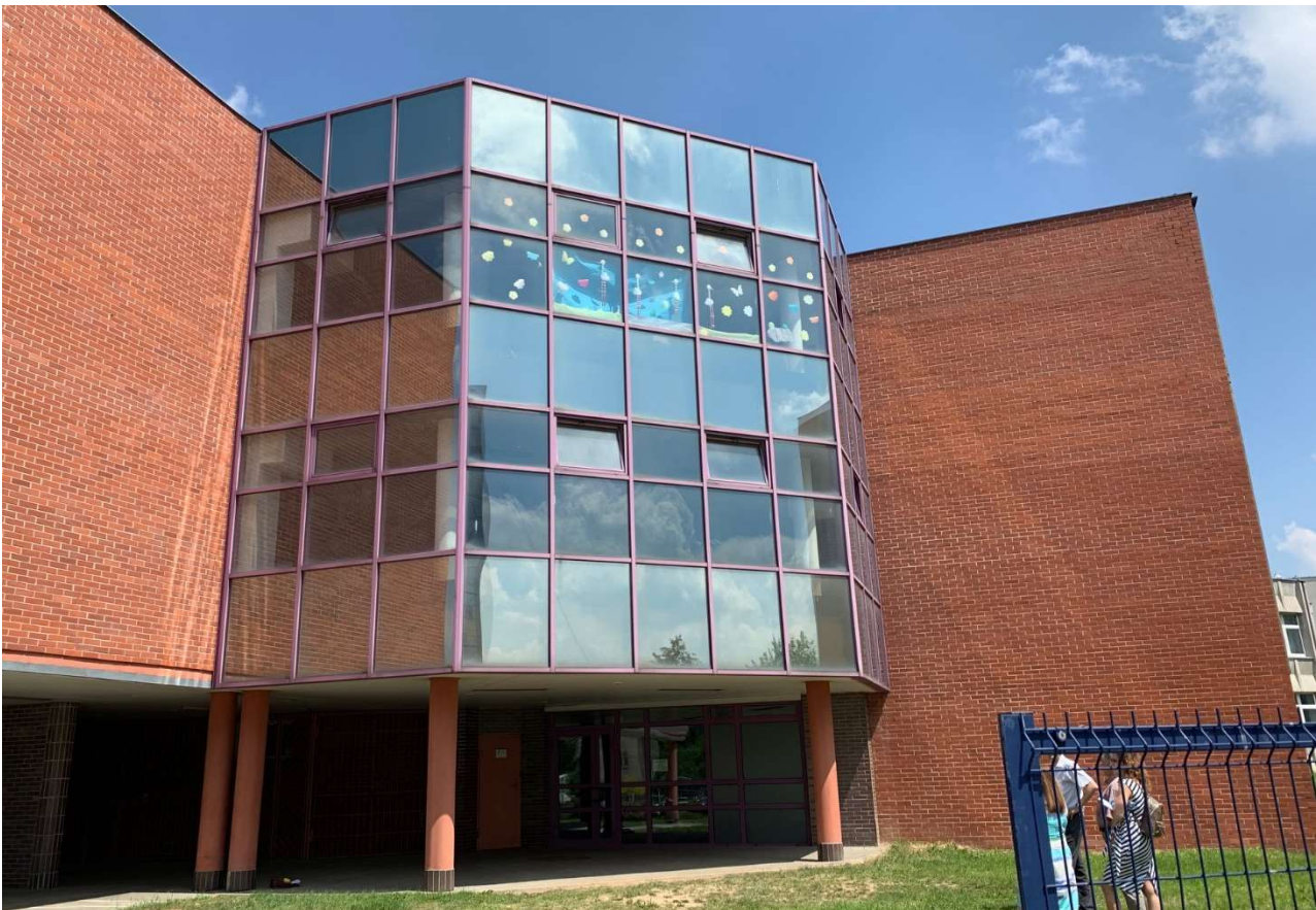
Figure 1: Polish Primary School, Dzierżoniów (Poland). The façade object of retrofitting
