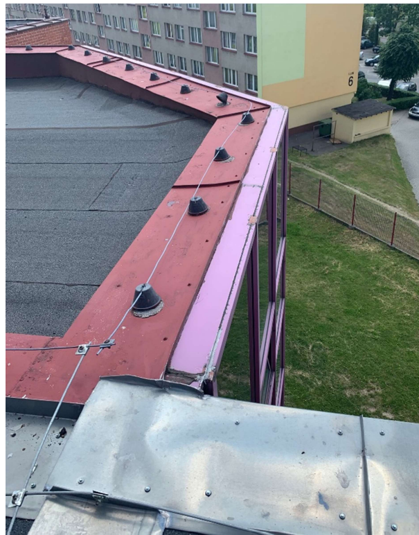
Figure 4: Interface between roof and façade
