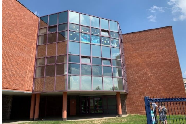
Figure 6 School façade before intervention – external view.
