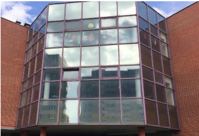
Figure 30 Façade view - before intervention
