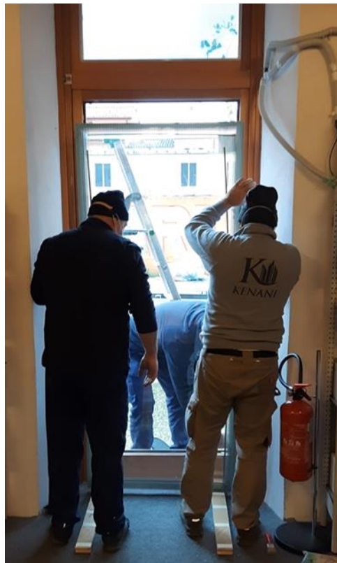
Figure 53 Placing the VIG.
