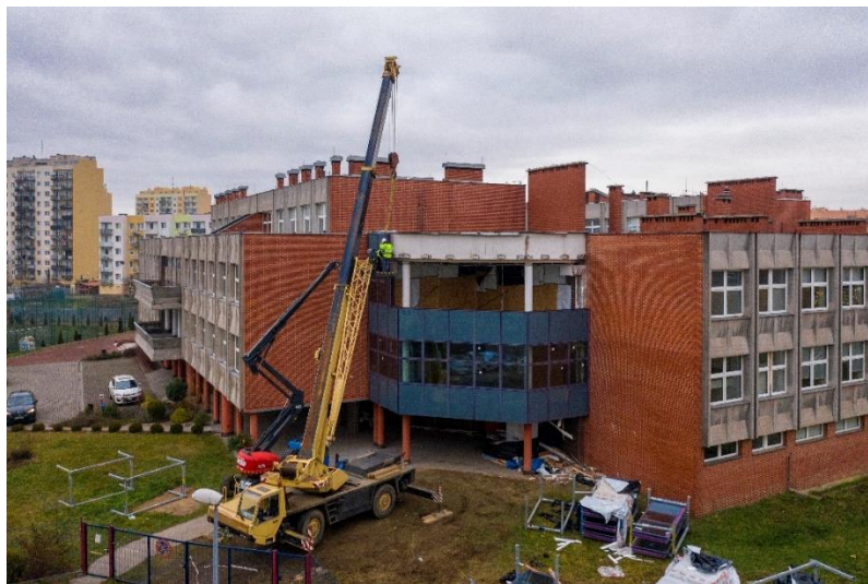
Figure 16 Crane used to lift facade modules
