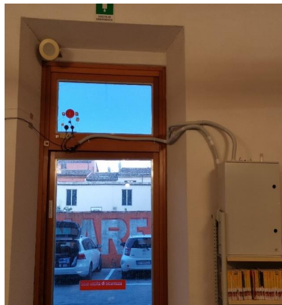
Figure 48 Library door - internal view.
