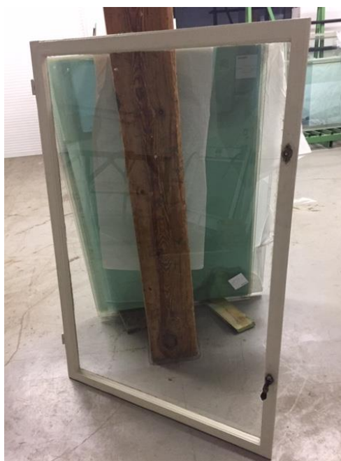
Figure 34 Window sash dismantled.
