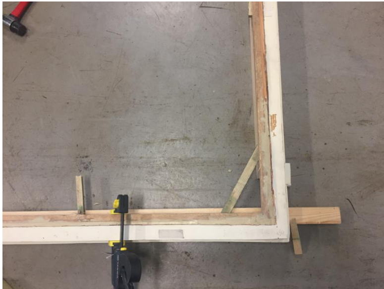
Figure 35 Old sash before renovation.
