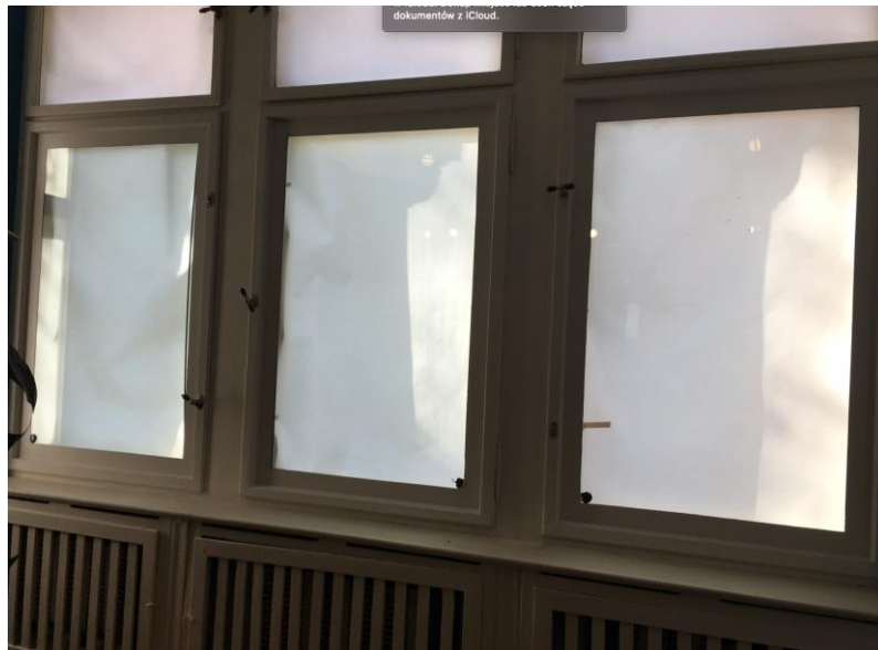
Figure 43 Window frames with VIGs - Internal view.
