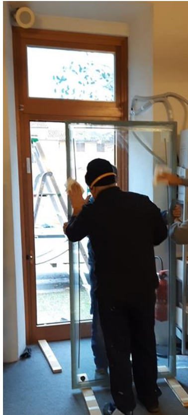
Figure 52 Preparing the VIG for installation.
