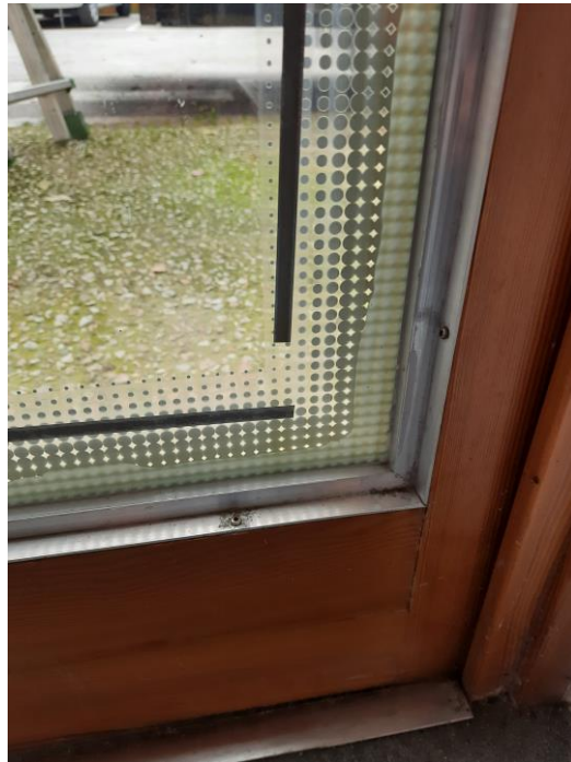
Figure 54 Glazing bead installed.
