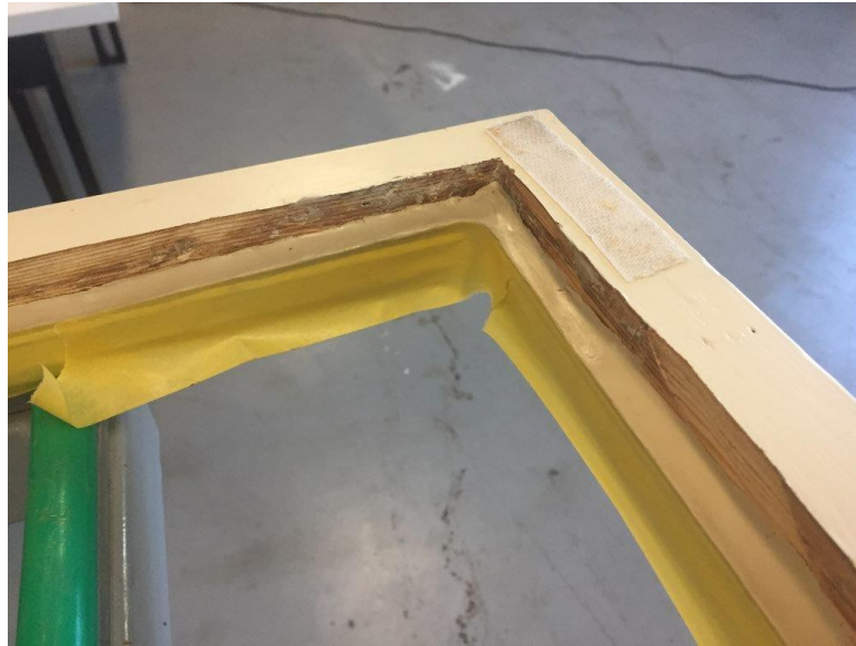
Figure 37 Application of the glazing putty.
