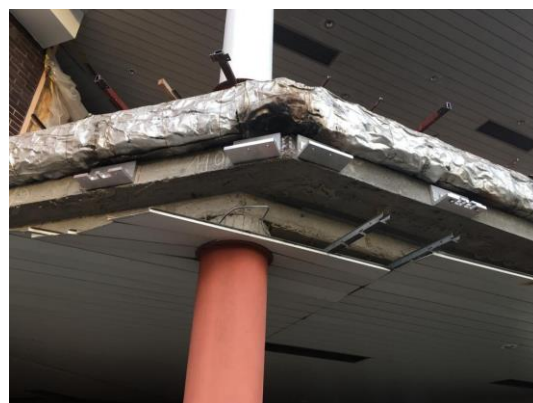
Figure 14 Brackets fixed to the slab – corner.
