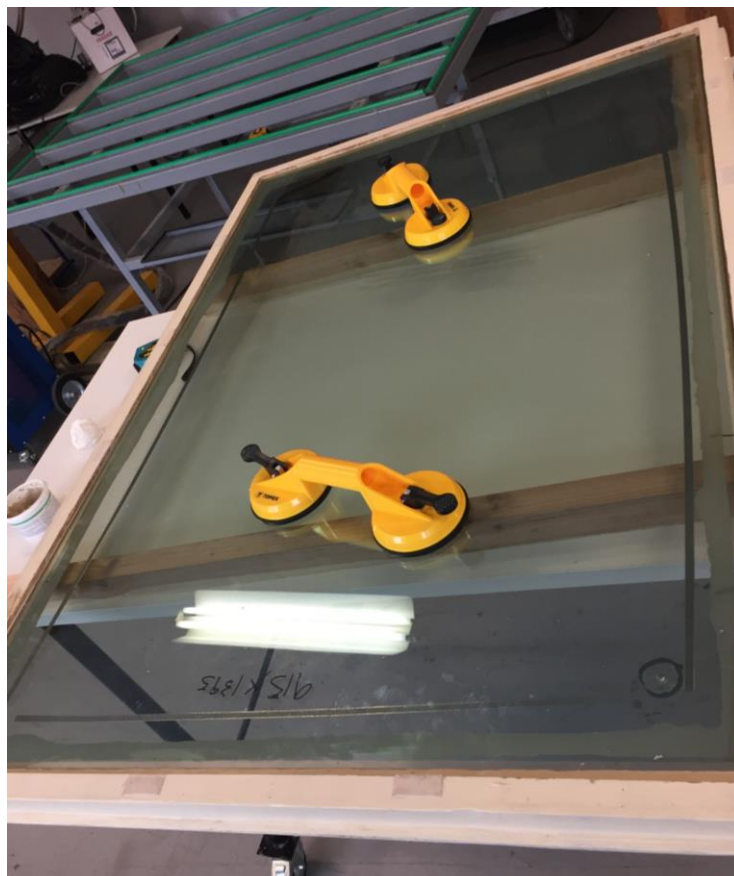
Figure 40 VIG glass inserting.
