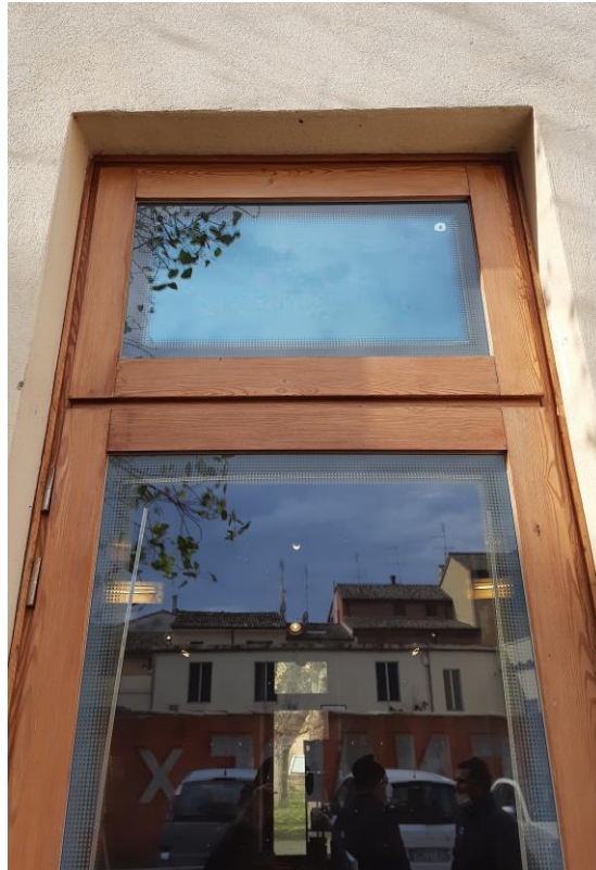
Figure 56 Door after intervention – external view.
