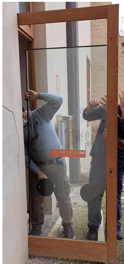
Figure 50 Old glass removing.
