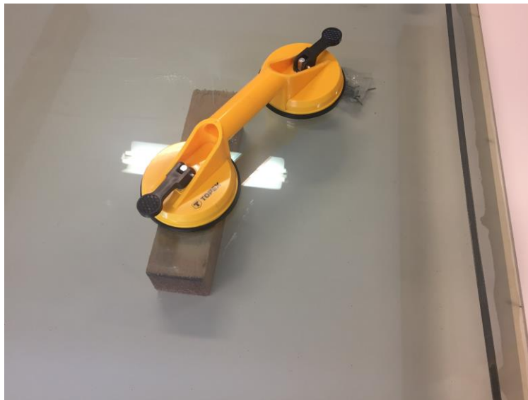
Figure 39 VIG glass to be inserted in the old sash.
