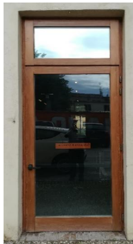
Figure 46 Library door external view- before intervention.
