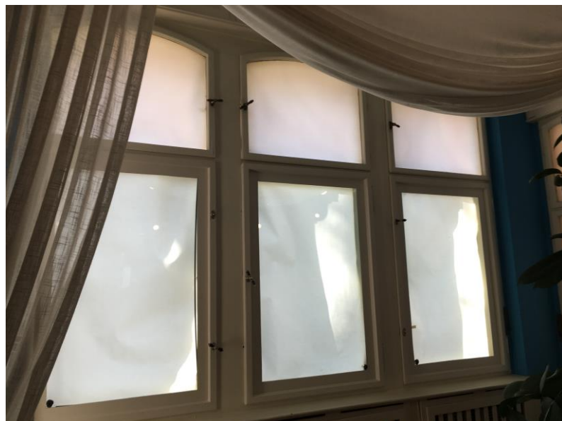
Figure 44 Museum windows after renovation.
