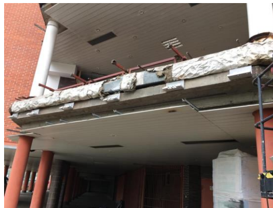
Figure 13 Fixing elements installation – brackets.
