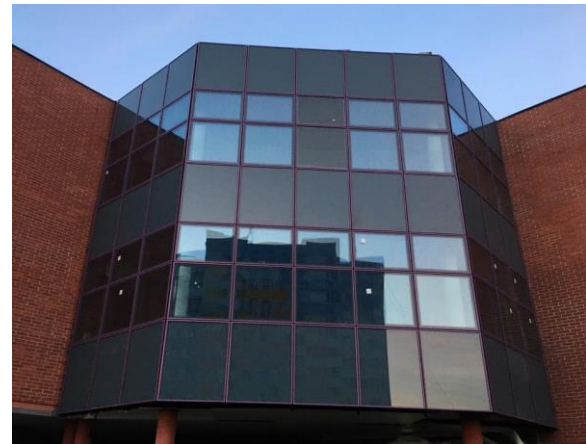
Figure 31 Façade view - after intervention
