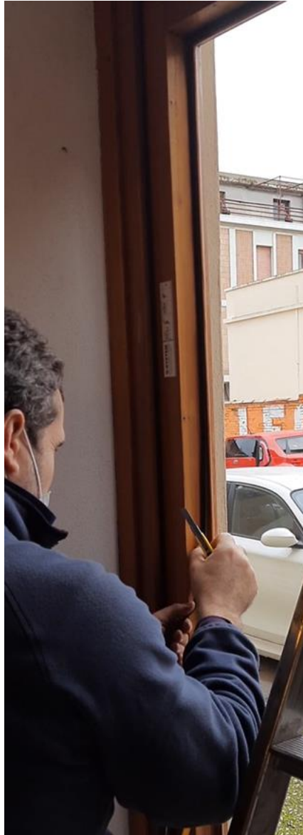
Figure 51 Cleaning the glazing area.
