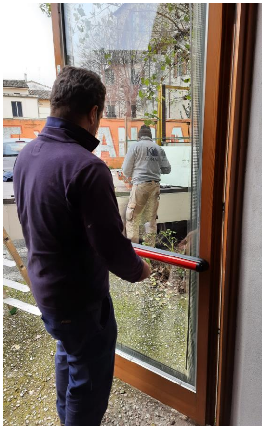
Figure 55 Handle installation.
