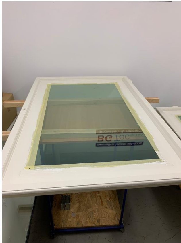
Figure 41 Window sash painted.
