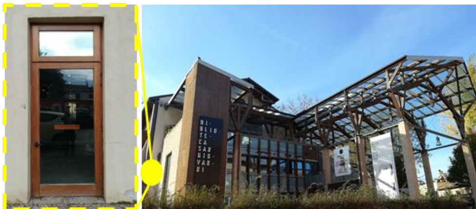
Figure 4.1 – San Giovanni Public Library: door-window [9]
