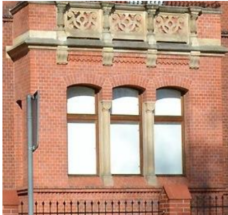
Figure 59 View of the existing windows – Dzierzoniow Museum
