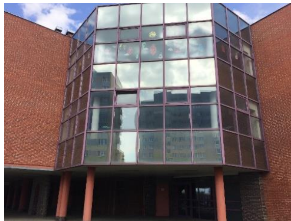
Figure 15 View of the existing façade in Dzierzoniow demo building
