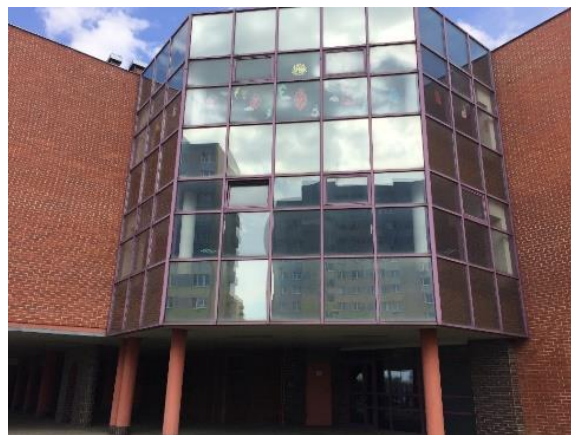
Figure 4 Existing façade – School external view
