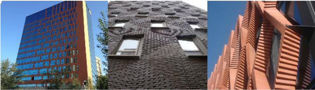
Figure 7-14 – Usage of ceramics in façade design
