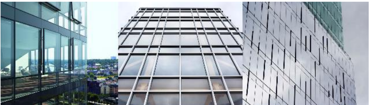
Figure 7-19 – Usage of glass spandrel in façade design
