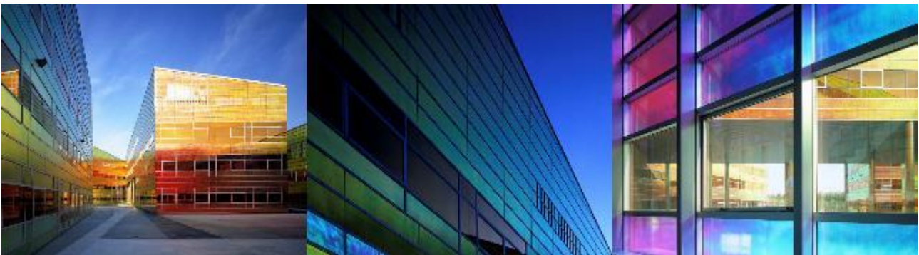
Figure 7-20 – Usage of dichroic foil glass in façade design
