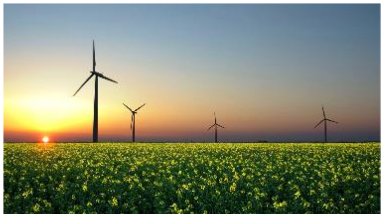
Figure 6-5 – Wind turbine farm
