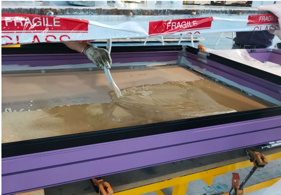
Figure 8 Spandrel part – foaming
