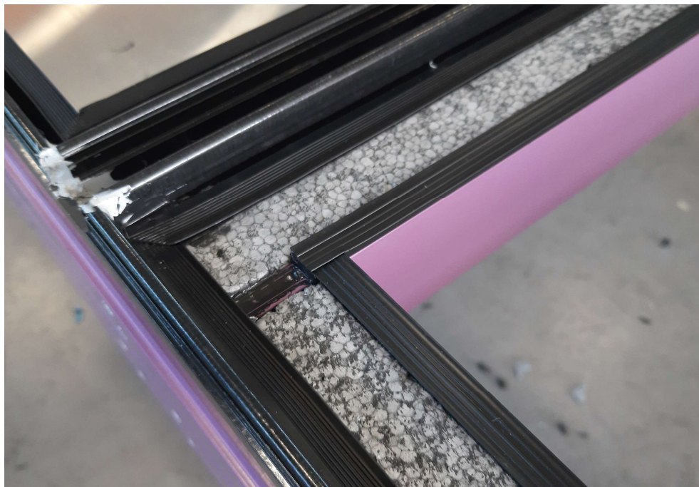
Figure 13 Vision part – EPS profile and gasket
