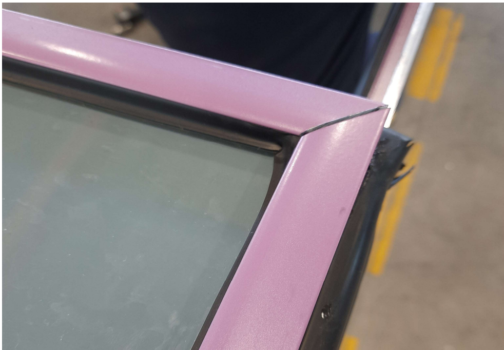
Figure 16 Mechanical restraint – gasket positioning
