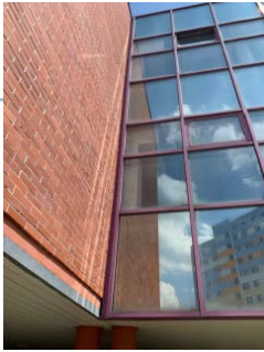
Interface between existing brick wall and façade
