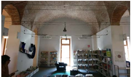
San Giovanni library and window chosen for monitoring
